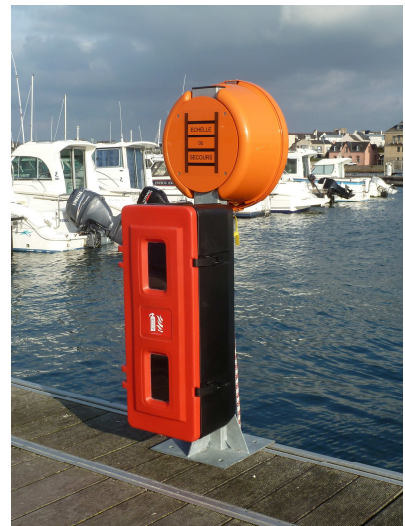
Pontoon ladder + fire extinguisher box
